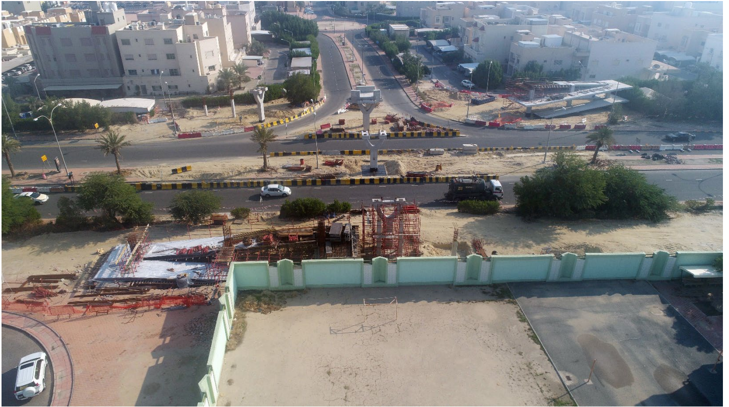
Foot Bridge 11 Works
