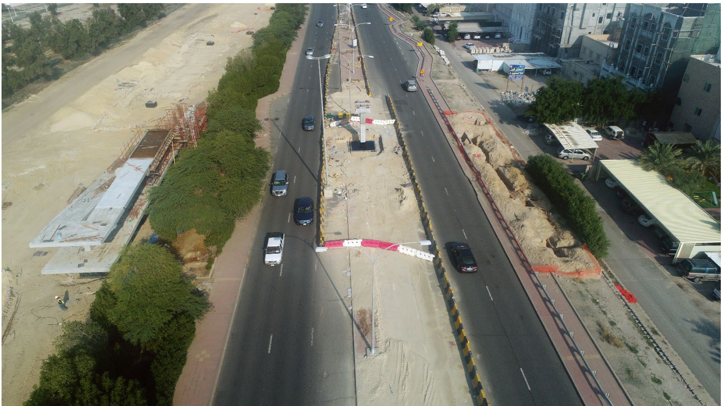
Foot Bridge 10 Works
