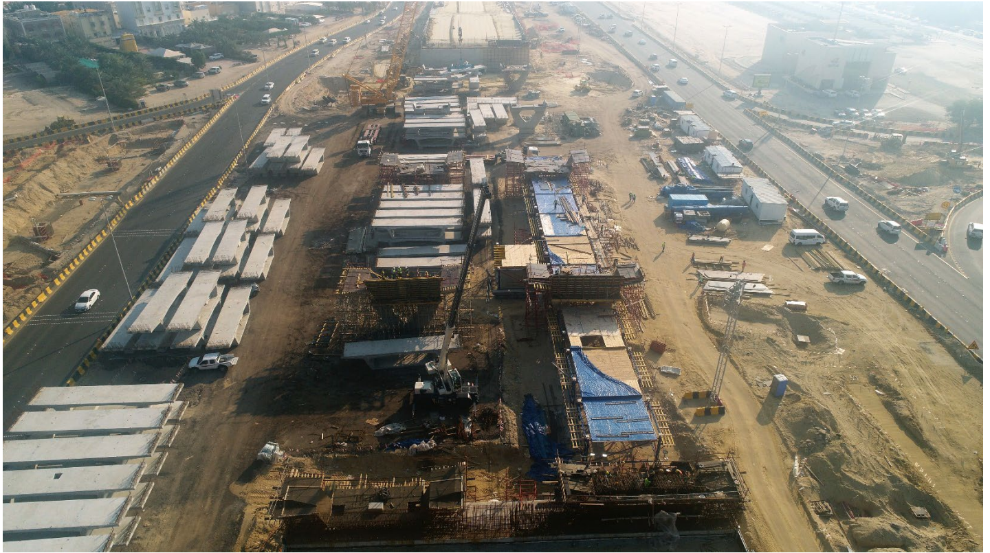
J26 – Mega Shore, Pier Segments & Abutment Segments Works
