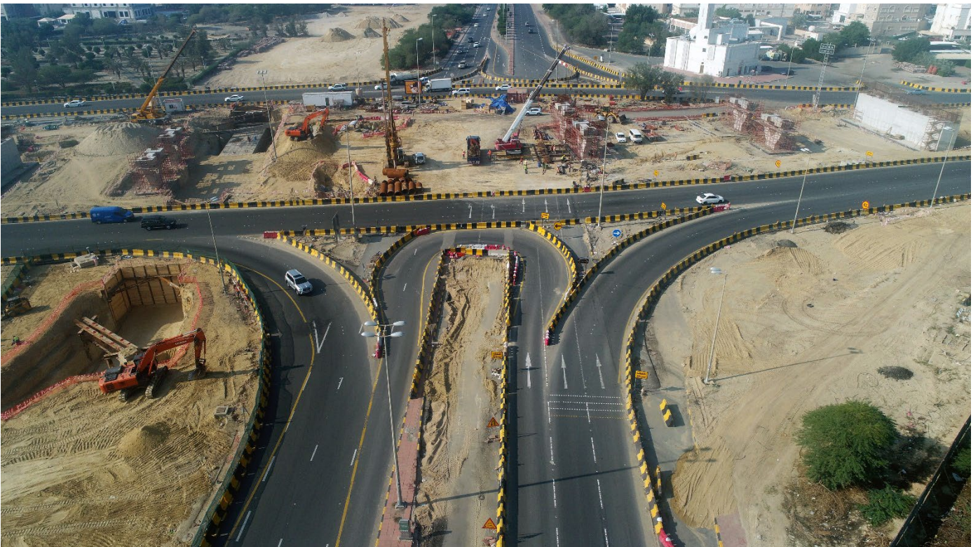
J16 – Bridges & Utilities Works
