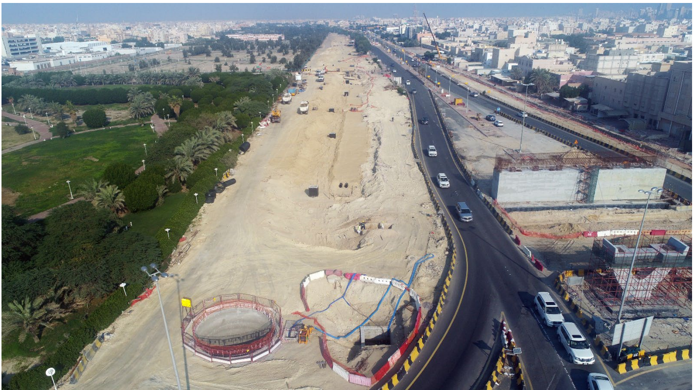
J18 – Micro-tunneling Shafts & Utilities Works
