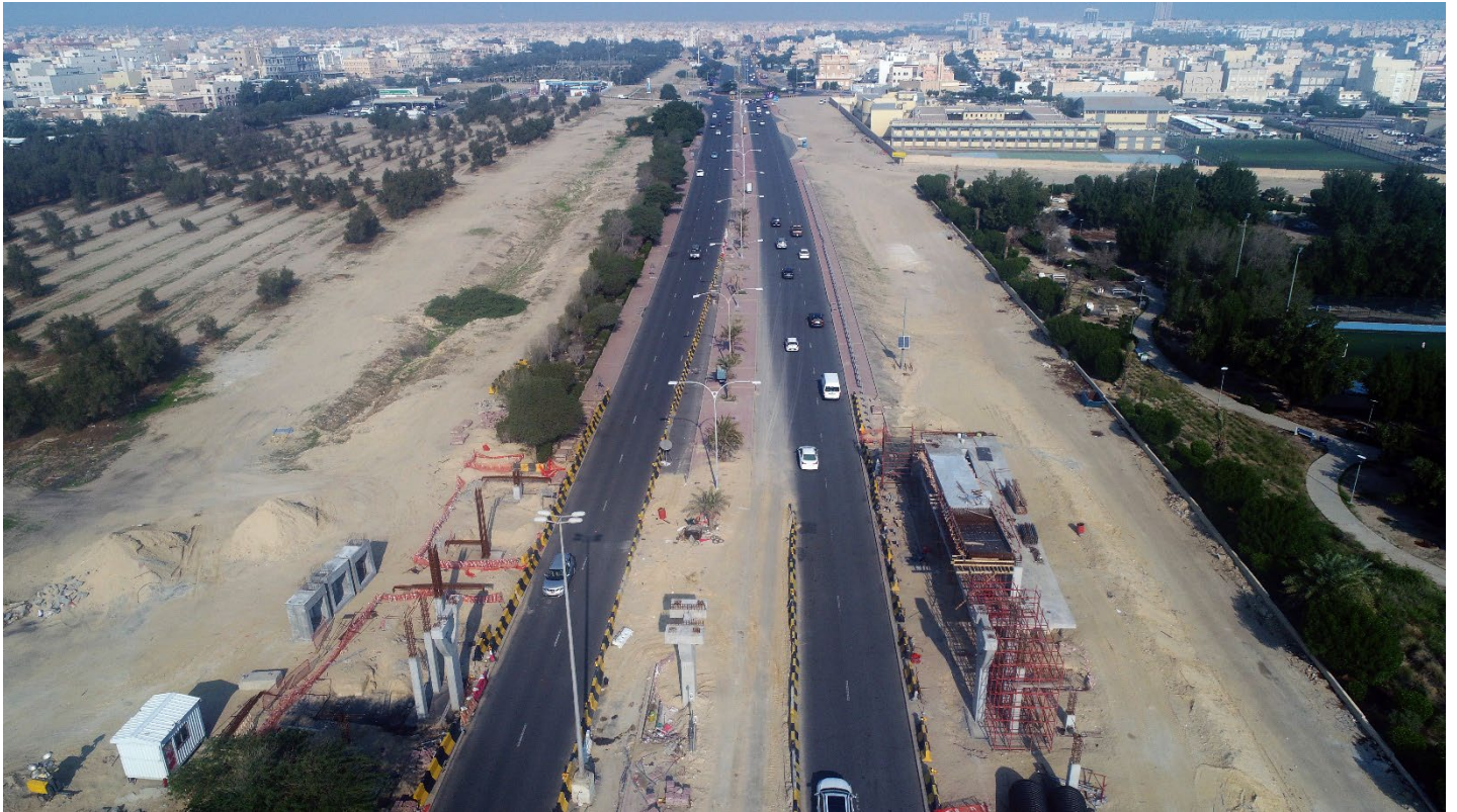
Foot Bridge 09 Works
