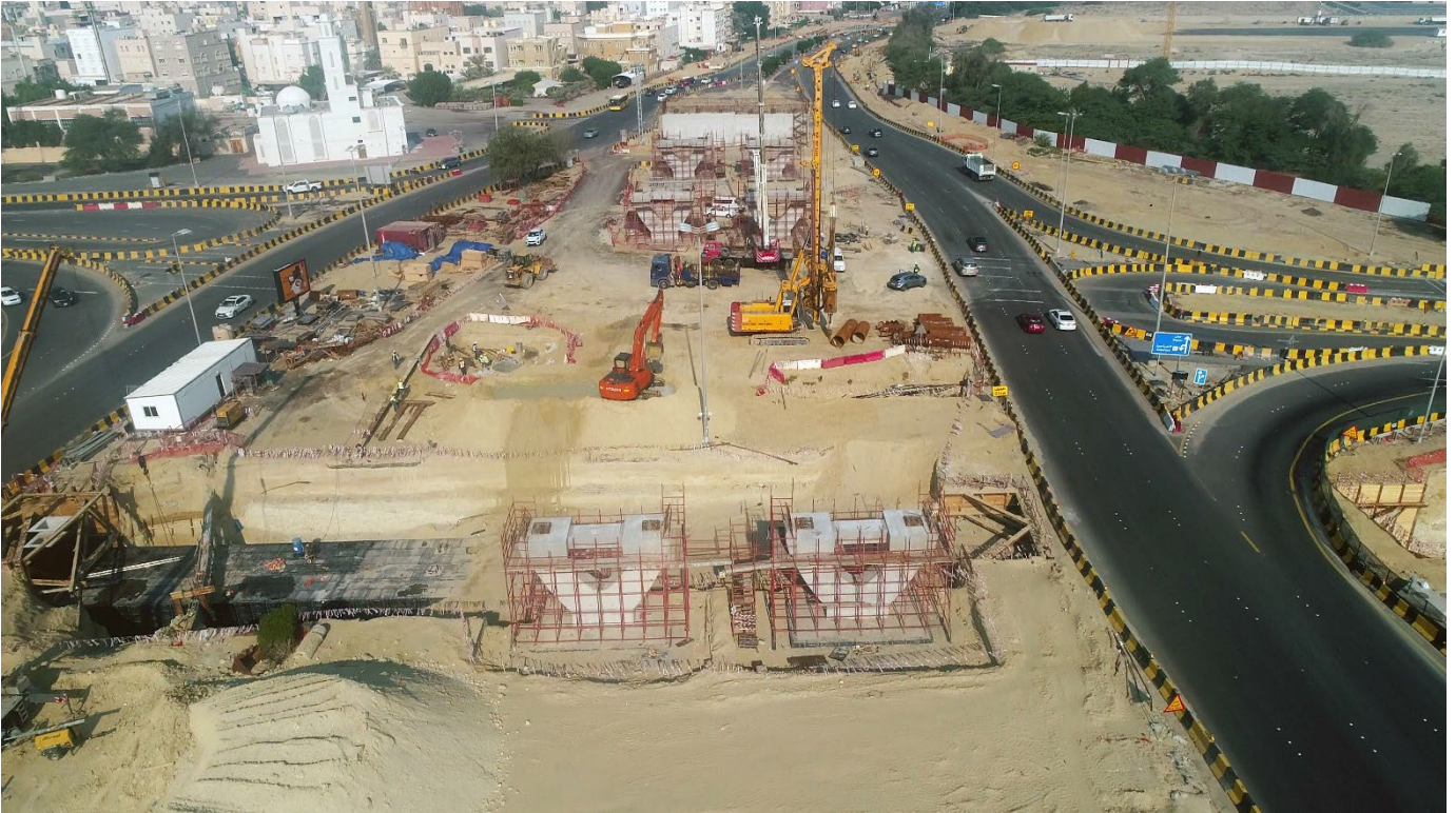
J16 – Bridges & Utilities Works
